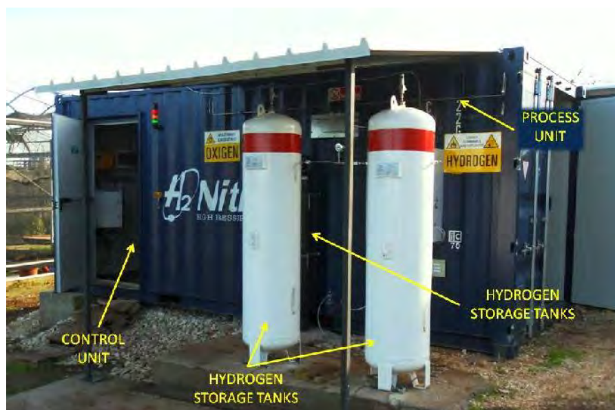
Figure 1. Plant external layout
