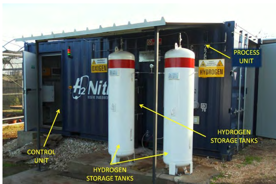
Figure 1. Plant external layout
